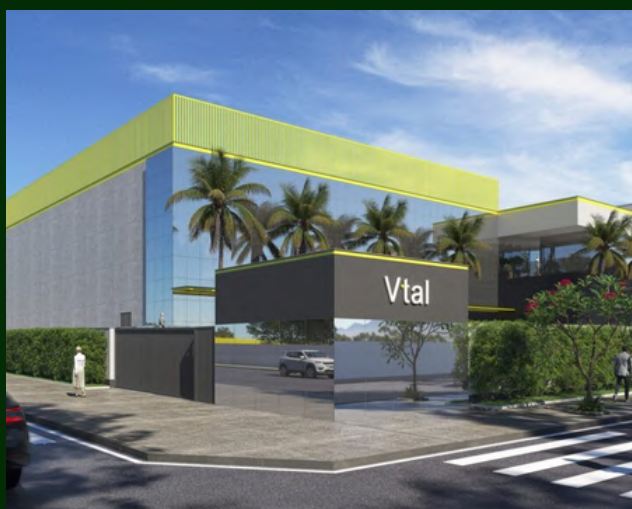
Data Center VTAL
